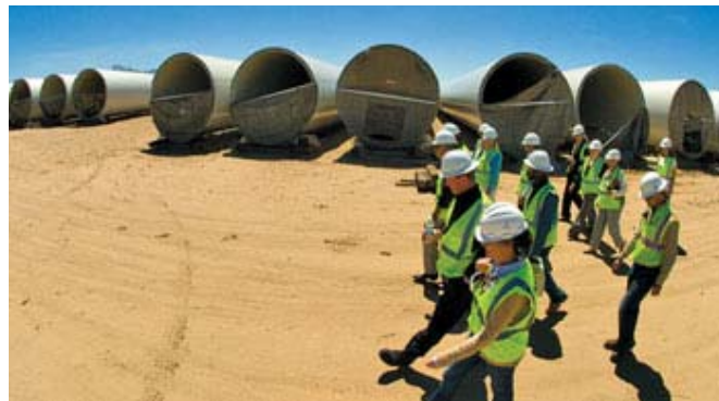
Utah's largest renewable-energy project, the Milford Wind Corridor, will be home to 97 wind turbines.
